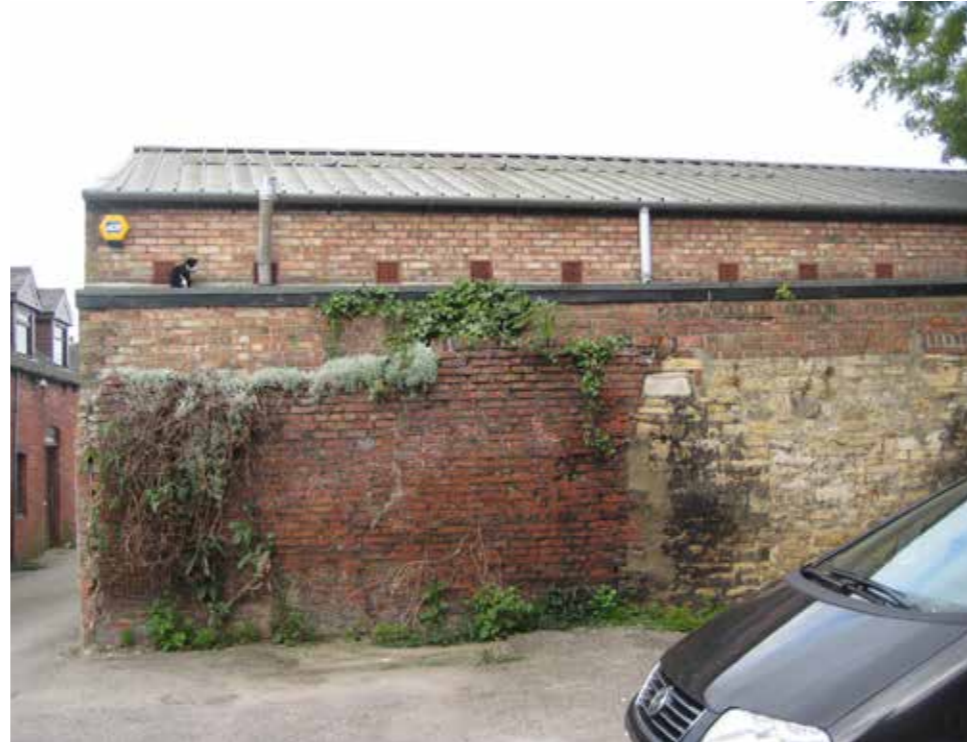
VIEW OF THE ORIGINAL BRICK AND STONE BOUNDARY WALL LOCATED TO THE NORTHERN BORDER OF THE SITE
