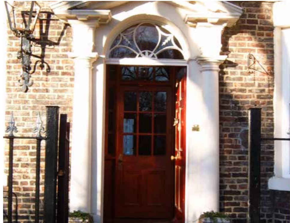
DETAIL VIEW OF THE MAIN ENTRANCE DOOR AND TUSCAN STONE PORTICO
