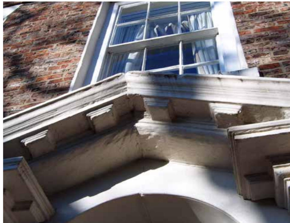
DETAILED VIEW OF THE MAIN ENTRANCE PORTICO
