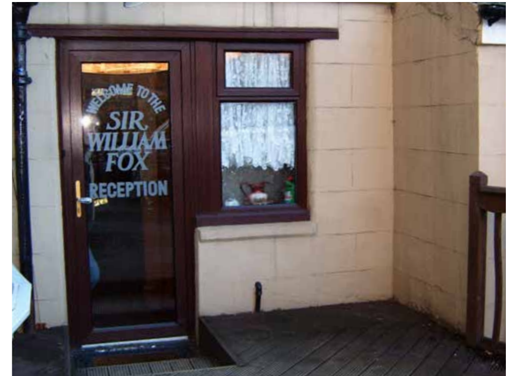
VIEW OF THE CURRENT ENTRANCE
